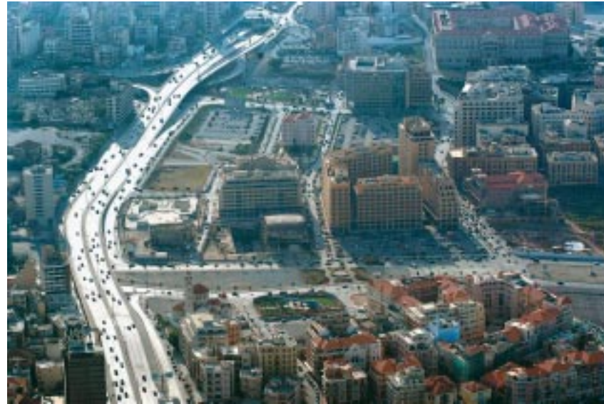
Southern view of the city center, with Fouad Chehab Avenue and the Martyrs' Square axis.
