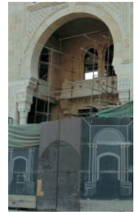
Stone repairs on the Grand Theatre façades.
