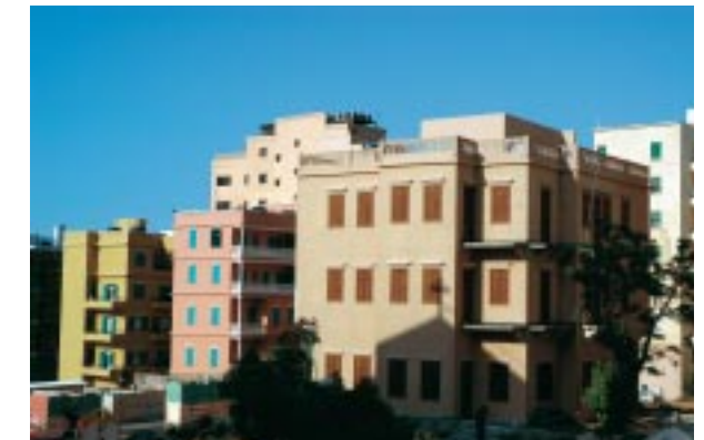
178 Saifi Village: interior façade rendering; restored existing building.
