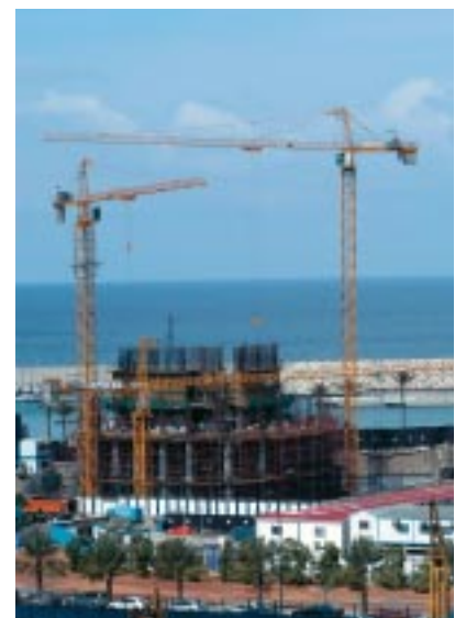
Marina Towers building site.
