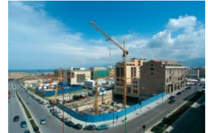
Building sites along Park Avenue.
